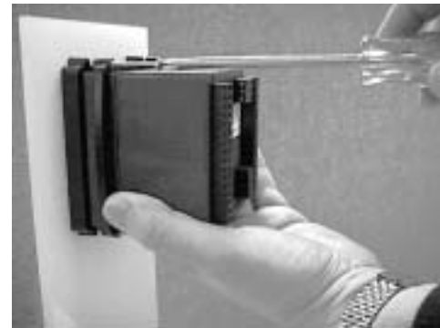
Figure 8.3c — Tightening the Screws.
